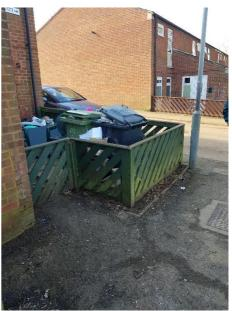
Fencing to the rear of the properties vary in height and styles. Some are rotten and/or damaged.
